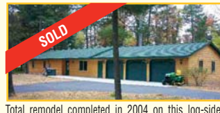
Total remodel completed in 2004 on this log-sided, 3BR, 2BA home. MBR w/MBA & WIC. LR has a gas FP & wood laminate flrs. Kit. has all new stainless steel appl. 4-season gazebo on back side of house. The 3-car att. gar. is insulated, sheet rocked, painted flr & blacktop drive. A must see at just $219,900 #135584 Call Ronn at 320-749-2326
